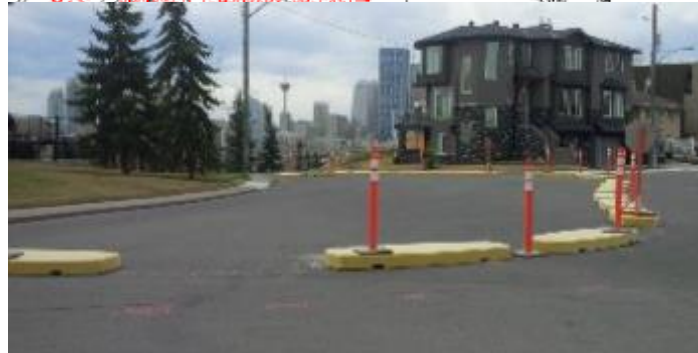
Traffic Calming Curbs Deployed in six hours with two staff Cost as placed $18,000
